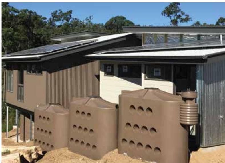
solar generation, with three of the rooves pitched to further maximise solar power generation. A total of 24 solar panels (Sunelec Pty Ltd) will be monitored for a 12 to 18 month period before the selection of a battery will be made.
