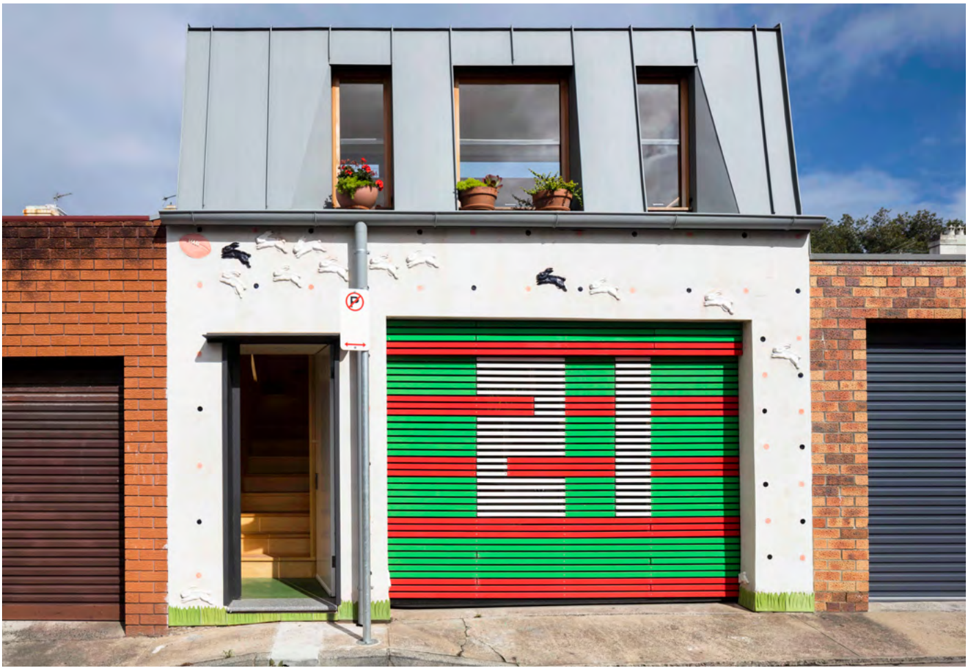
Architect Peter McGregor's garage-top studio sits harmoniously in its laneway context. "As the need for density and intensity of use grows, the 25-square-metre footprint is an increasingly important model for the fine-grained pedestrian city," he explains. The garage door was designed to show support for the local NRL team.
